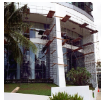
Scaffold set up to paint the exterior main lobby
