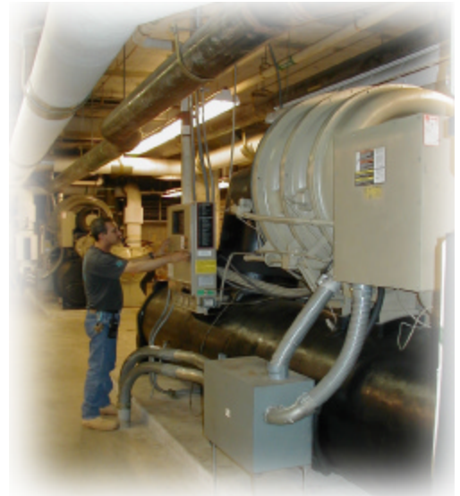
One of two Centrifugal Chillers
